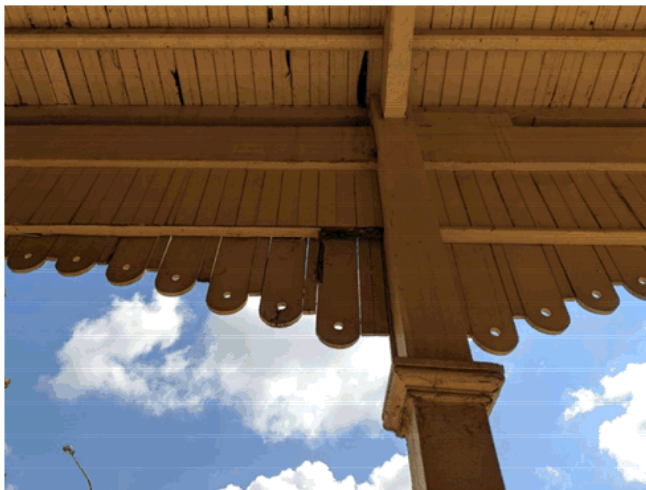
Picture 5 Note that the framing to the valance panel is rotten and will need repair/replacement. Note also the damaged floor boards
