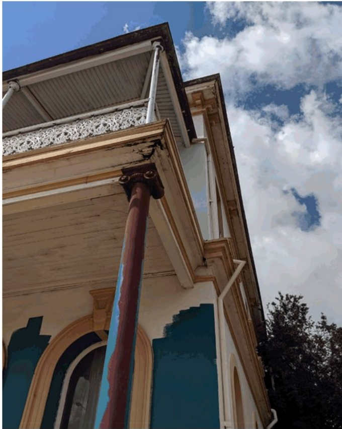
Image 4 water overflows from the top corner before it can get to the downpipe. The dp may also be blocked
