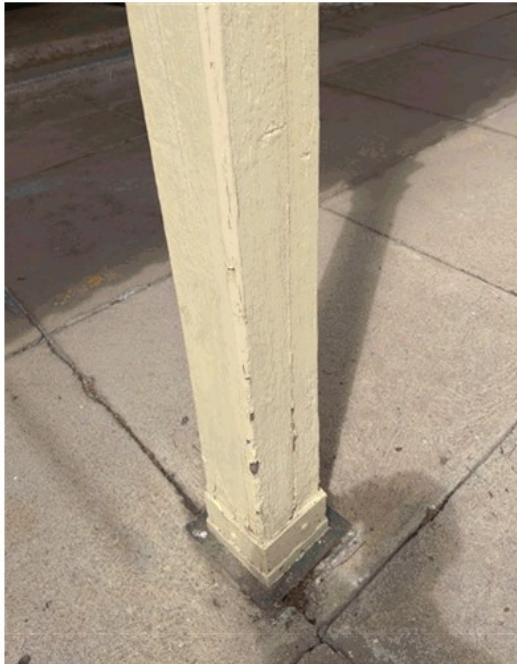
Picture 2 Damage not evident in post 2 but steel base needs replacement
