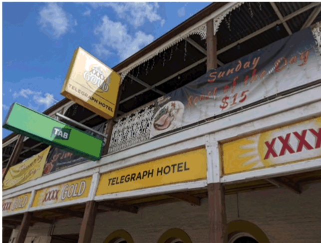
Photograph 5 General view of the verandah and the cast iron. Note the stop chamfers on the posts and beams and the recessed panels.
