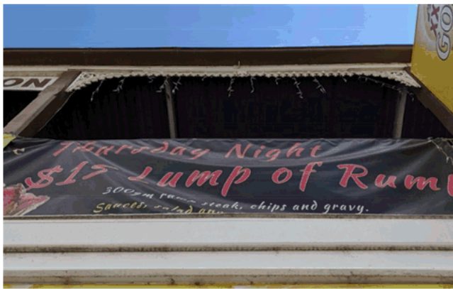
Photograph 14 Upper cast iron elements to be re-installed with missing pieces fabricated by Wagga Foundry
