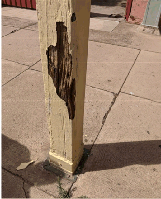
Picture 1 A seriously damaged area to the eastern posts with what appears to be termite tracking aggravated by damp
