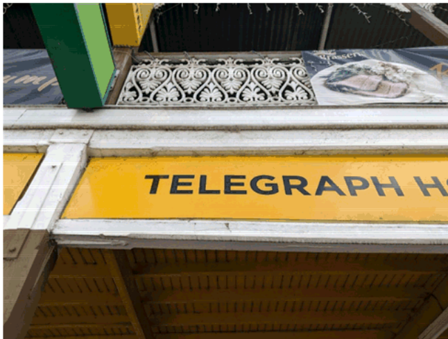
Photograph 6 Note the inset sign panels and chamfered details on the timber framing.
