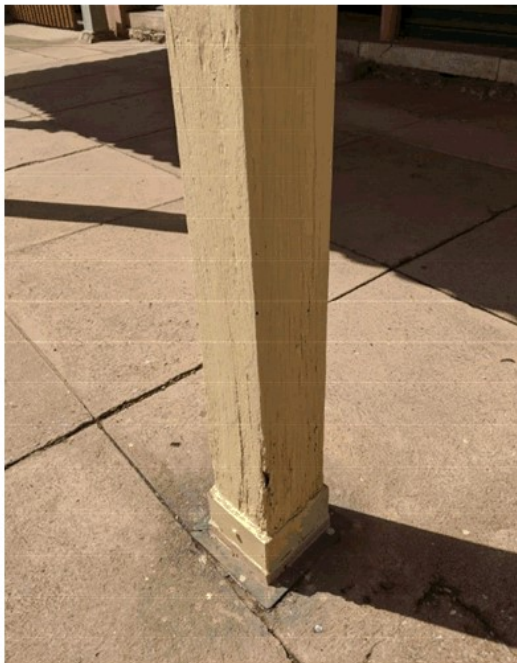
Picture 3 Minor damage near base 3 with splice possibly required
