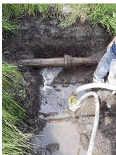
Trunk water main repair
