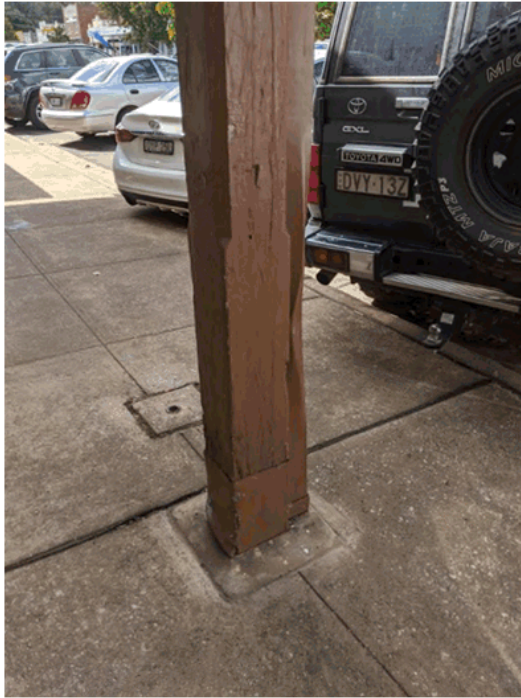
Photograph 4 Post bases to be replaced with concealed stirrups. Note the start and stop points on the chamfers to the posts
