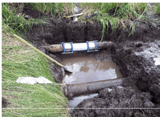
Trunk water main repair
