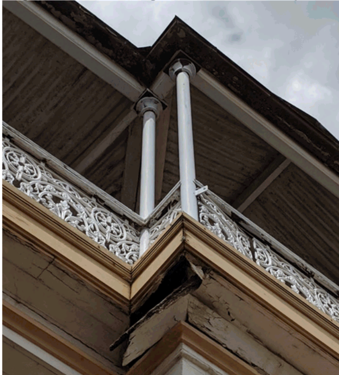
Image 8 An almost complete loss of lining boards due to unconstrained water. It is likely that the structure supporting the cast iron posts and roof above these will have been affected.
