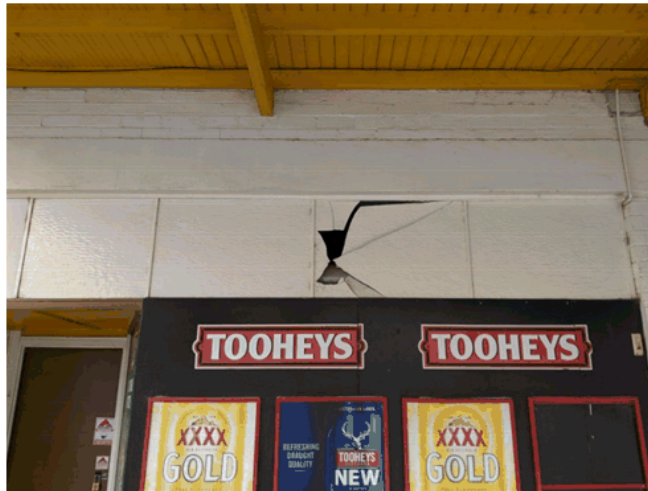
Photograph 8 Obscure glass panes to be reinstated where damaged
