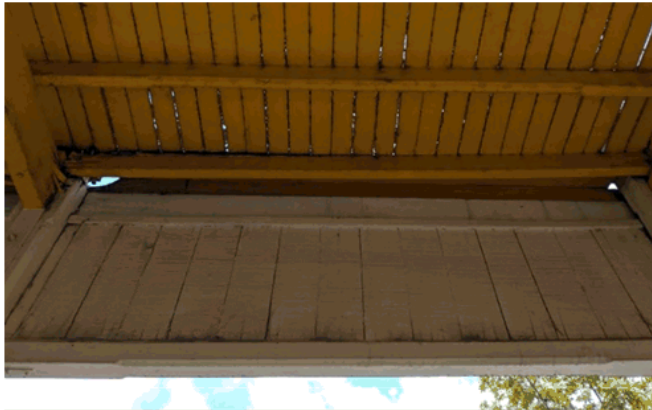
Photograph 13 Board facing behind sign panel area
