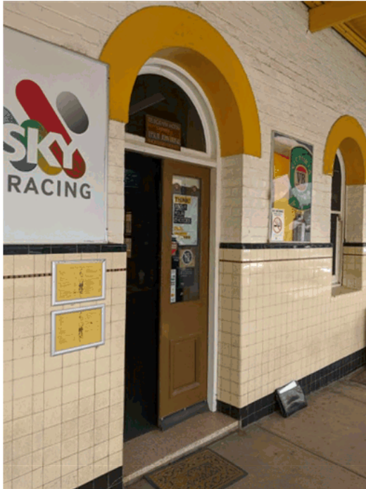
Photograph 2 Tiling, brickwork, door/window frames, doors and rendered details.
