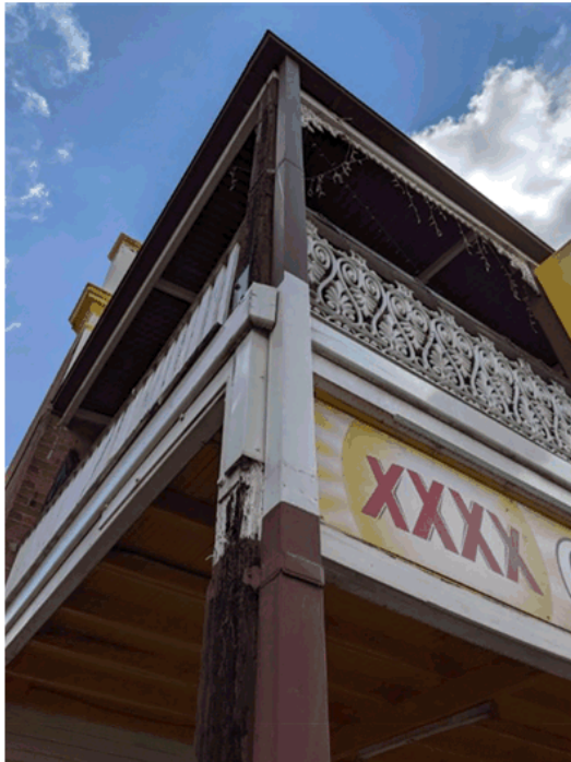
Photograph 10 New downpipes to be painted 90mm pvc and side balustrade to be new cast iron to match original. Confirm with Council that 1m is the required height of the handrail and 125mm the maximum space through the balustrading.
