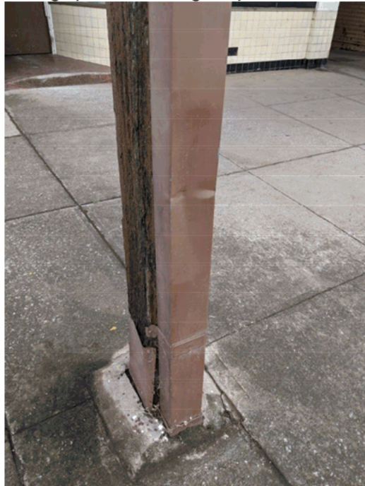
Photograph 9 Post base and downpipes to be clamped using traditional steel brackets to posts
