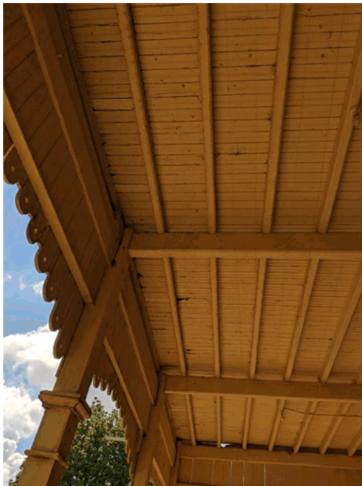
Picture 6 Note that insufficient drainage appears to have damaged some timber flooring and timber trim details
