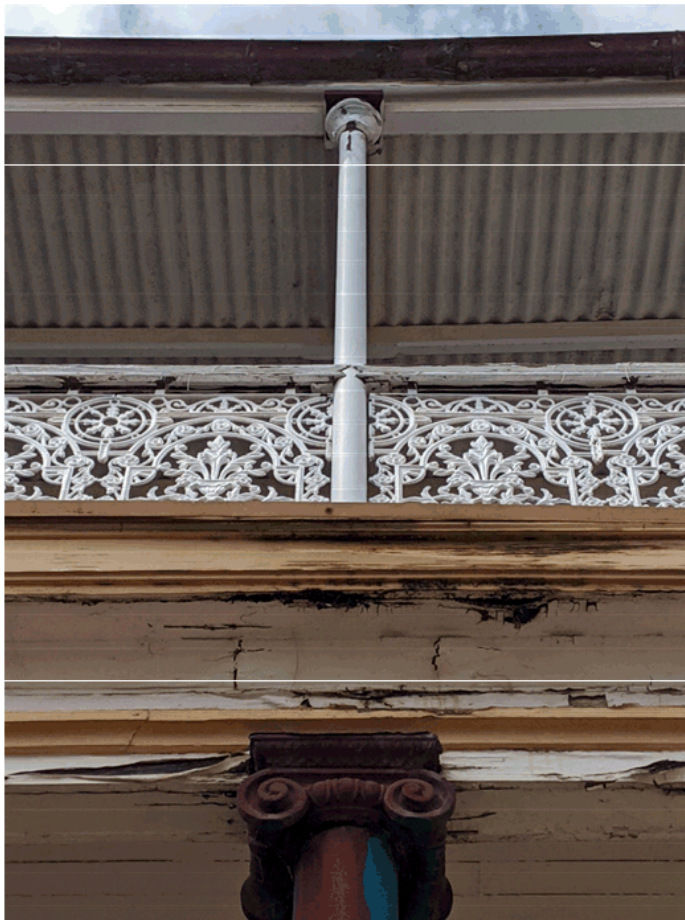
Image 6 The extent of the damage is clear at the major structural elements which support the verandah
