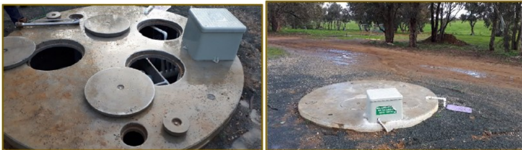
Commissioning of multi-chamber enviro septic unit
