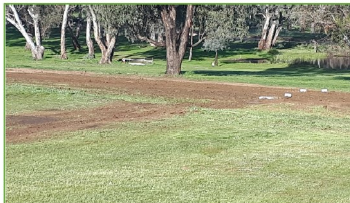
Molong Showground Septic -New reln trenches, larger capacity grease trap, new junction port & drainage lines
