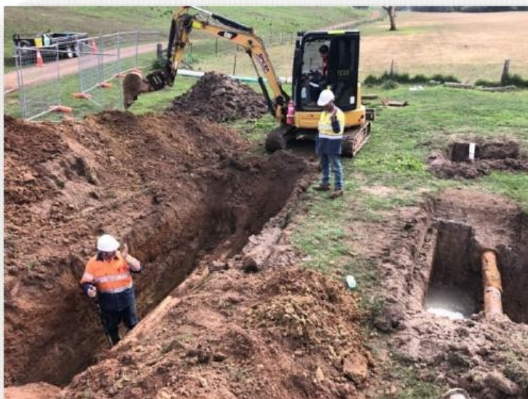
Image Above: 'Peter's Pit' - Where the Molong Creek Dam raw water main meets the Borenore dam original line
