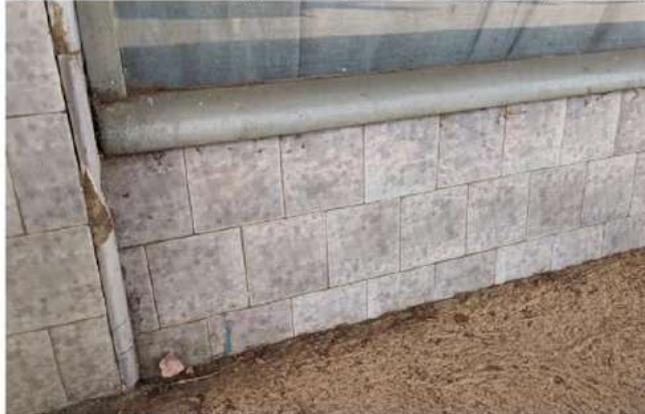
**Figure 4** The ceramic tile facing and nickel shopfront - significant element. Generally intact, these finishes are intended to be weather protected and will decay rapidly if there is no verandah or awning.
