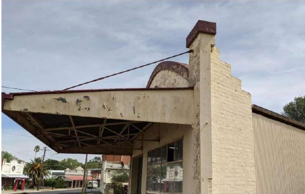
**Photo 2** Side view to illustrate the shed to the rear clad in painted galvanised iron, the brick return and the rendered façade with suspended awning
