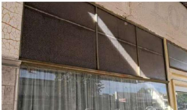
**Figure 5** The upper portion of the shopfront including the nickel shopfront frame, stippled glass to the hamper panel area and special scrolled nickel details to the frame - significant element.
