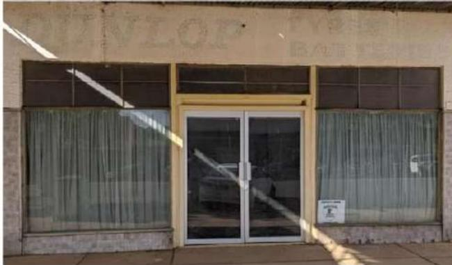
**Figure 6** The full shopfront element, noting the replacement door set. The corporate branding is showing through on the painted area above the top lights.
