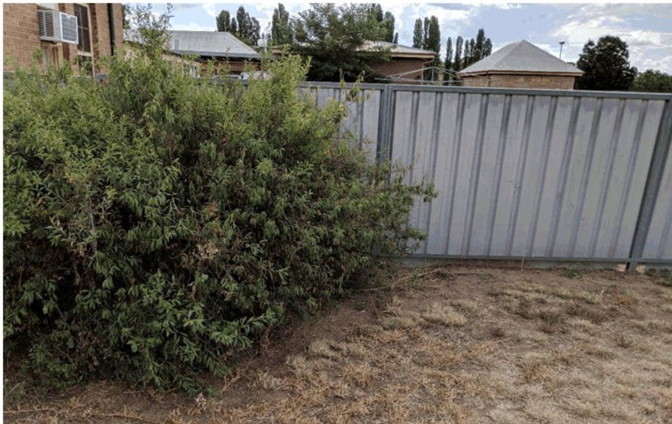
Image 18 Recommendations: replace steel deck fencing with traditional corrugated steel sheet fencing Metroll Corodeck in Windspray
