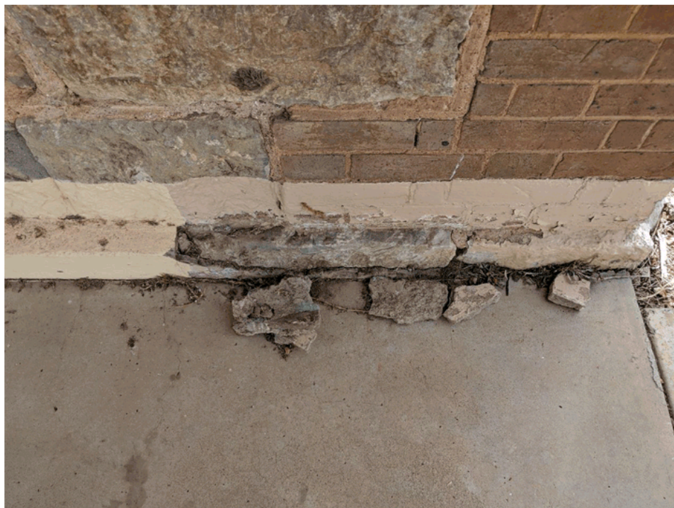
Image 36 Damaged render to building base on front verandah to be restored and paint removed from above that base.
