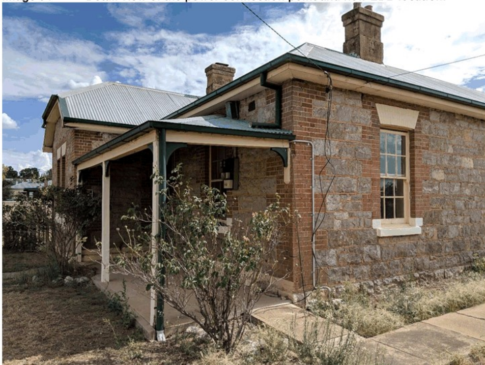
Image 35 Key elements to be painted. Location on the side wall for the new/replacement electrical switchboard. Galvanised standard steel cabinet with Painted 'Windspray' conduits
