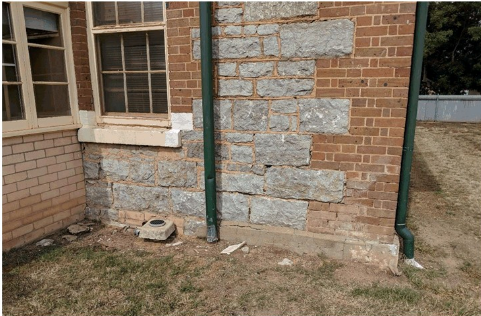
Image 10 Recommendations: Brick and stone repair and perimeter ground treatment as above. Colours for downpipes to match walls. Paint cream brickwork to match colour of existing brick in the quoins.
