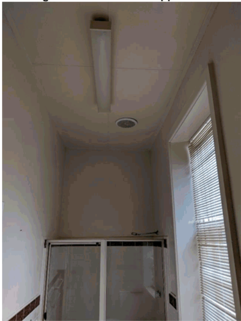
Image 27 Recommend retaining existing tiling, shower and vanity. Replace ceiling fan with in-line ducted unit and roof mounted flue and radiant heat panels from Devex using comfortline panels. Ensure window opens for natural ventilation.
