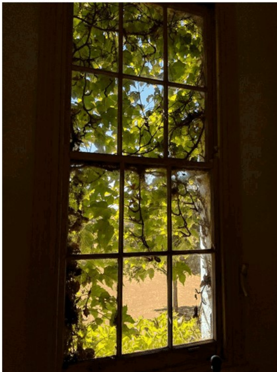
Figure 8 A typical double hung sliding sash window
