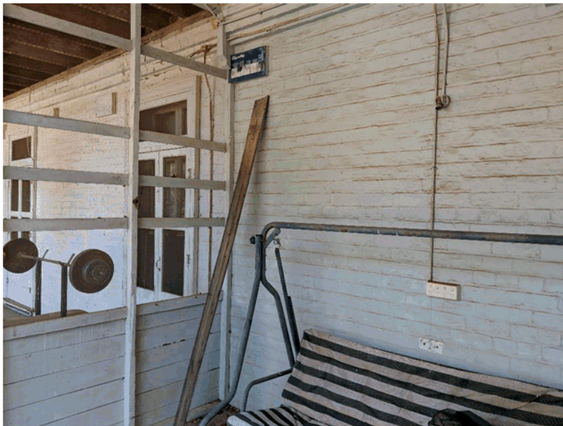
Figure 26 View of the painted external ground floor walls in the area previously enclosed. Experimenting with Peelaway or Soy-gel removers would be worthwhile to reinstate portions of the face brickwork.
