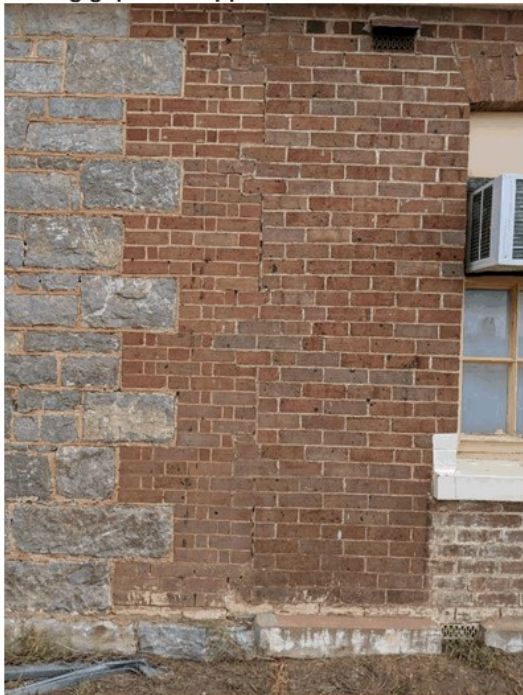
Image 16 Recommendations: Restore lime based mortar pointing and seal all gaps and joints. Do not render over exposed granite foundation course.
