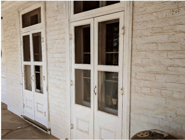
Figure 23 Typical French door sets to the front East Elevation.
