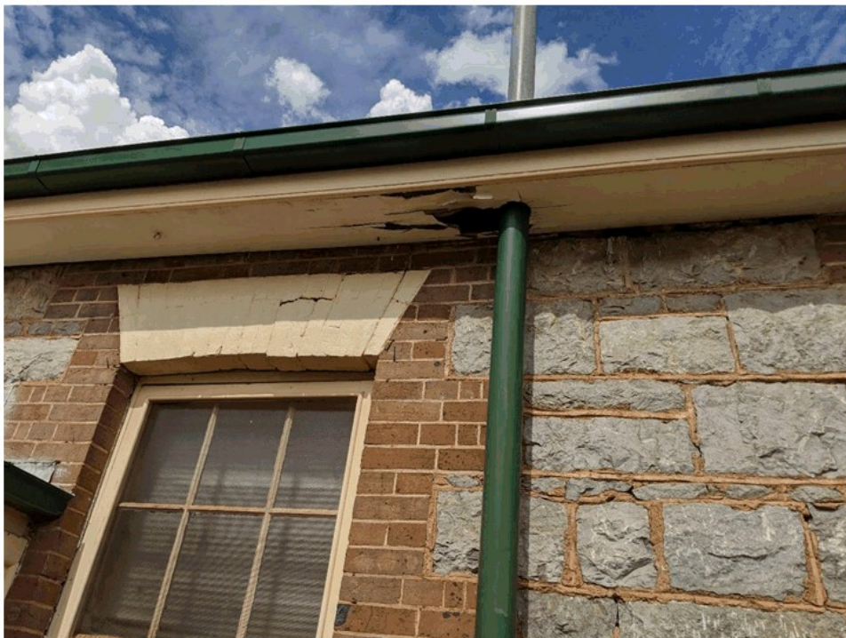
Image 9 Recommendation: Replace damaged eave with drilled - ventilated eave sheet. Repair brick lintel course – Brad Jenner.
