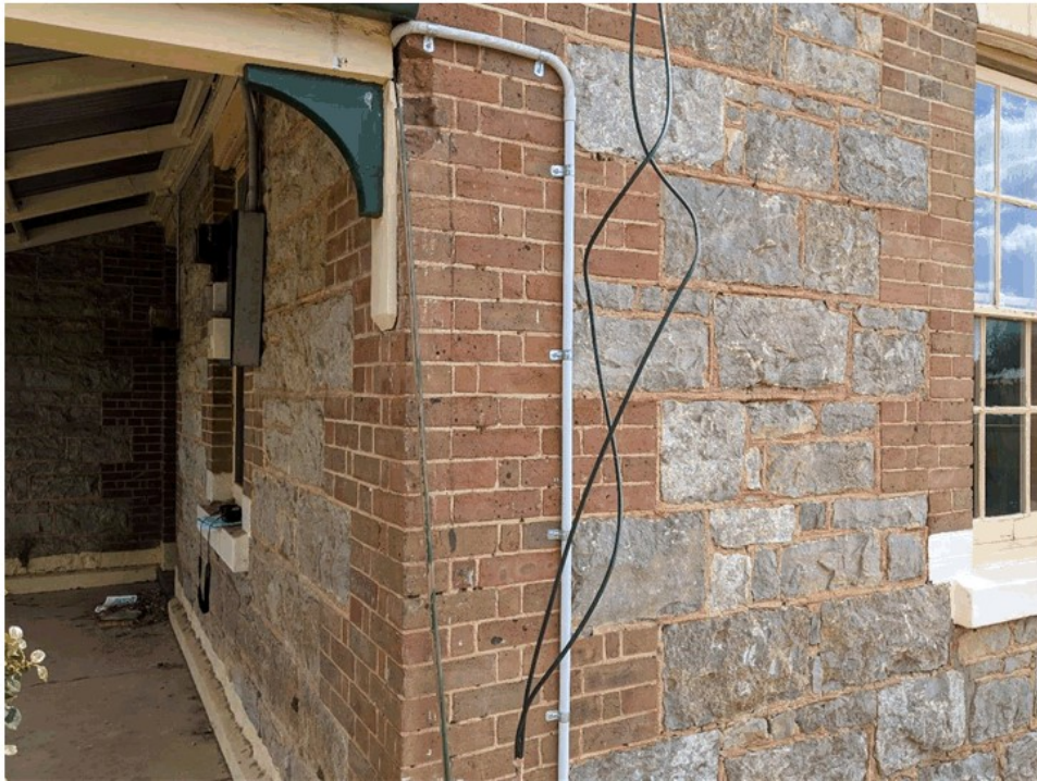
Image 34 Detail view of the power connection point and new EDB location.
