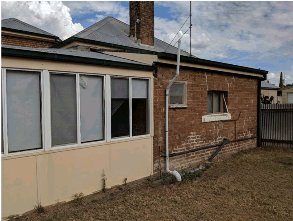
Image 13 Recommendations: Brick pointing repair with lime based mortar and perimeter ground treatment. Paint downpipes to match brick colour.
