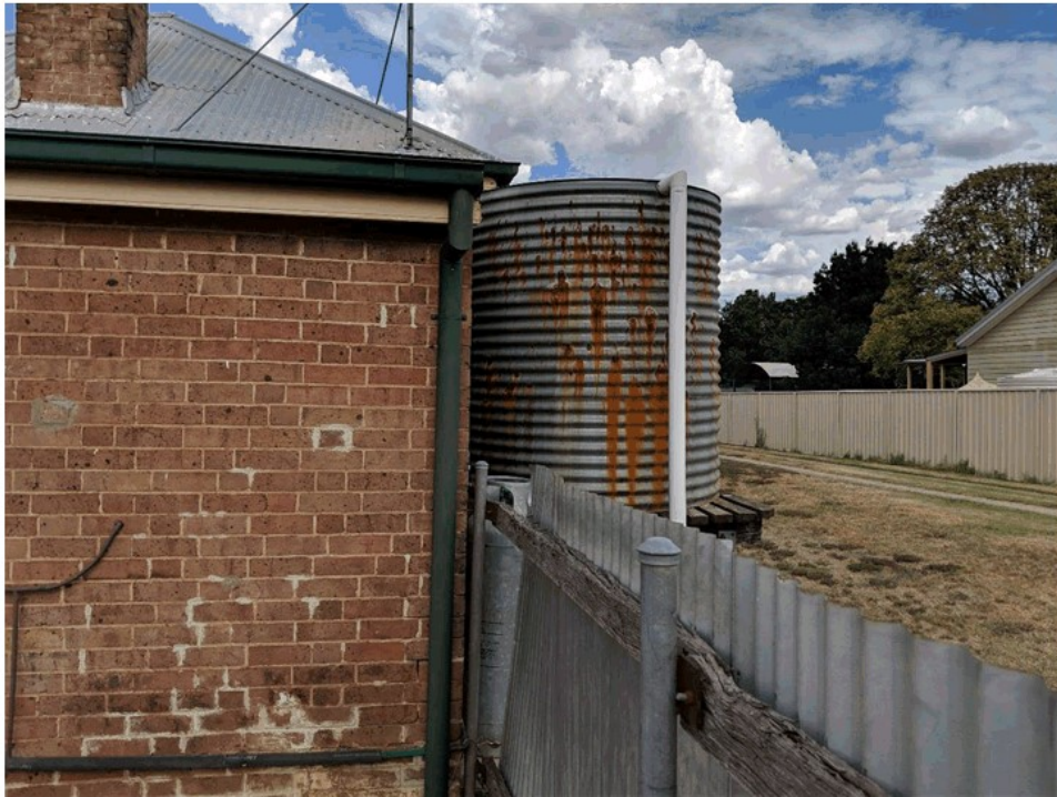
Image 12 Recommendations: Metrol Corodeck fencing only if existing steel sheeting requires replacement, replacement traditional galvanised steel corrugated rainwater tank and lime based mortar re-pointing by a skilled professional as noted.
