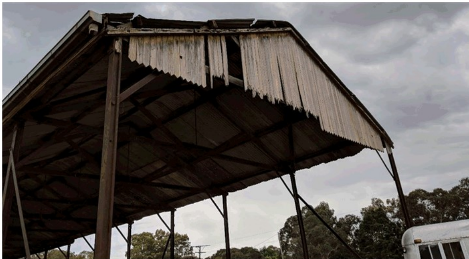
Photograph 2 The north elevation of the grain shed – timber and roofing elements for repair
