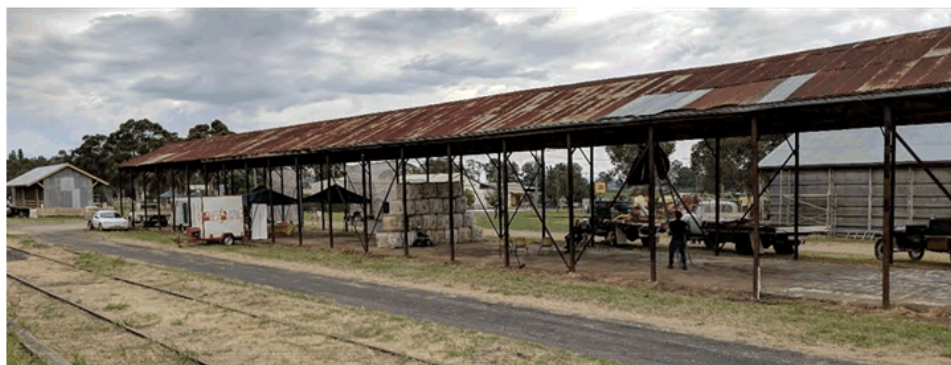
Photograph 1 General view of the East Elevation, noting the condition of the roofing with previous substitute sheets, missing gutters and temporary provision of electrical services.
