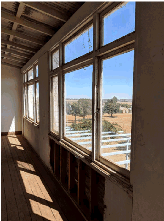
Figure 14 View of the two window panels which are subject to consideration for either reinstatement to a suitable form or a removal with the provision of replacement weatherproof floor.
