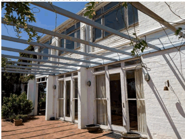
Figure 3 View of the north Elevation, noting the two bays of enclosed space comprising the kitchen and dining spaces. As this space is to be retained the first floor will either need to have a weatherproof floor when the open area is restored or the first floor space will need to be enclosed using traditional details evident in the following photos.
