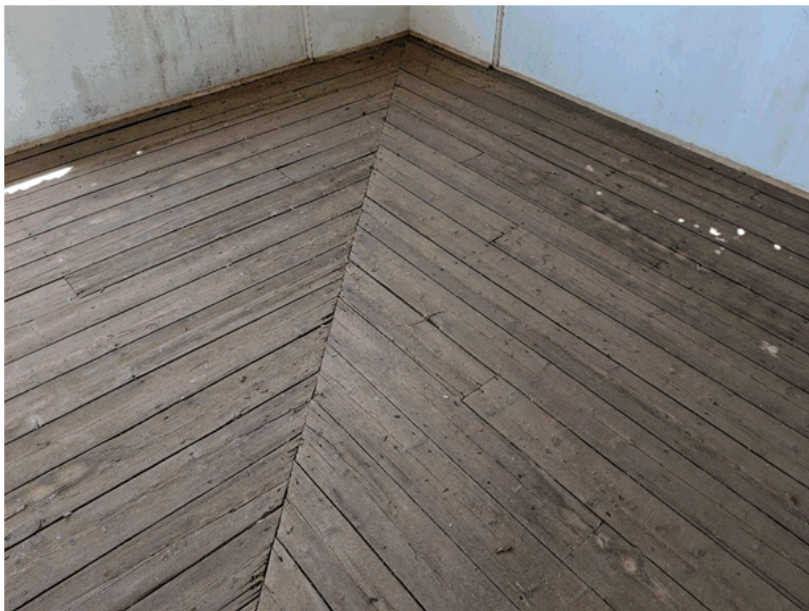
Figure 10 View of the verandah floor at the NE corner showing the original boards. The mis-matching may indicate that the flooring was modified or replaced at some stage. Traditional verandah flooring ran at right-angles to the building so that water would run-off the 1.40 slope. The condition of the boards has been protected by the last 60+ years of the enclosure.
