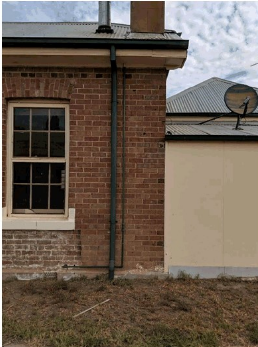
Image 15 Recommendations: Ground perimeter treatment, paint scheme and sealing gaps with applied timber moulds.
