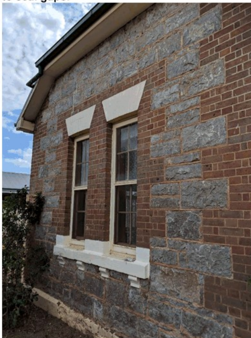
Image 20 Recommendations: Restore damaged timber and soffits. Refer new paint colour scheme
