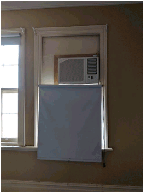
Image 26 Recommendations: Restore window after replacing AC. Consider floor standing AC unit instead of upper wall mounted unit as part of split system.
