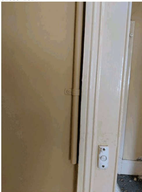
Image 29 Exposed and painted conduit acceptable. Power points by Tradco heritage antique copper
