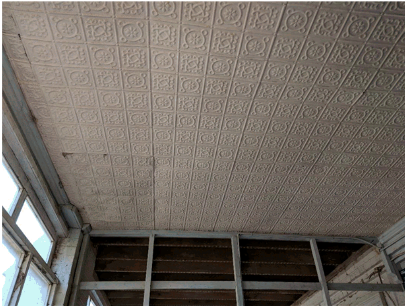
Figure 27 Pressed metal ceiling to the former enclosed ground floor room within the southern verandah.
