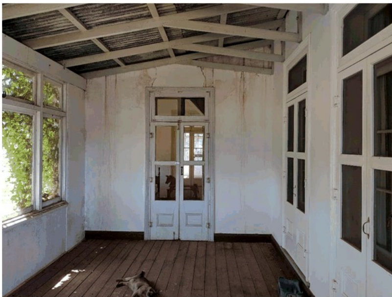
Figure 12 View to the NE corner of the existing enclosed verandah noting the original French door set, the bedrooms to the right and the modified braced roof structure and overlapping galvanised iron roof sheeting. The roof braces detract and
