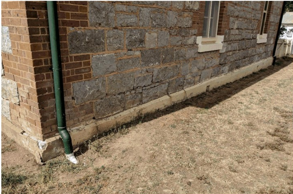
Image 8 Recommendations: Masonry restoration by Brad Jenner Orange, plus ground treatment to replace 1200mm wide topsoil strip to 150mm with 150mm compacted roadbase laid to fall away and base render reinstatement & paint.
