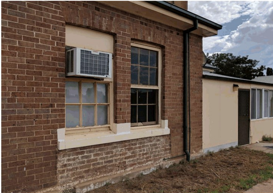
Image 17 Recommendations: Clean and restore face brick finish using Peelaway or Lets Clean soy gel. Restore traditional window following AC removal. New paint colour scheme. All downpipes painted to match brick colour.
