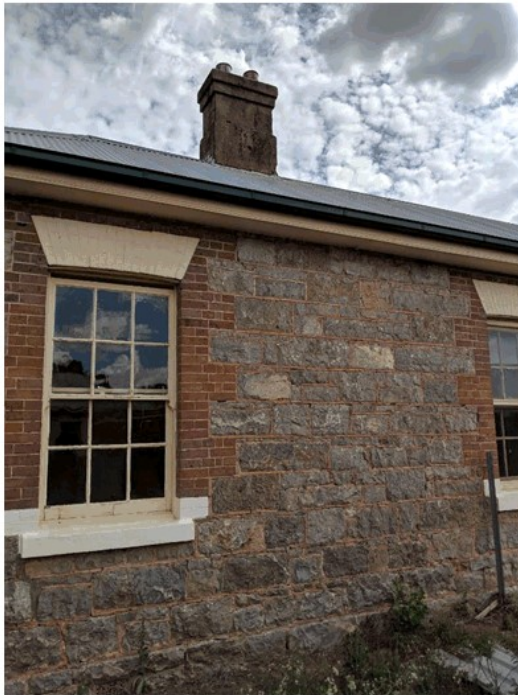
Image 19 Recommendations: Ground perimeter: replace earth to 150mm deep to 1200mm width with compacted roadbase and steel perimeter edge at 1.40 slope away from walls. Essential to control damp/moisture. Fit \frac{3}{4} round mould at eave wall junction to seal gaps.
