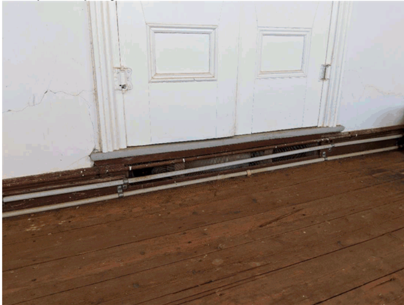
Figure 13 Typical French door set, noting the step down, the gap and the random service conduits.
