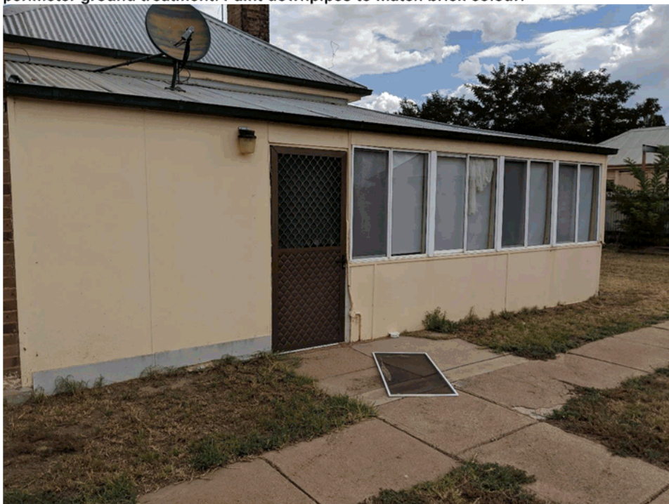
Image 14 Recommendations: New paint scheme and compliant steel security screen door to replace aluminium decorative screen door.
