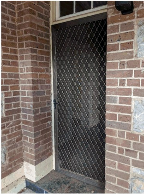
Image 23 Recommendations: Replace screen door with compliant steel framed secure-mesh or similar security door
