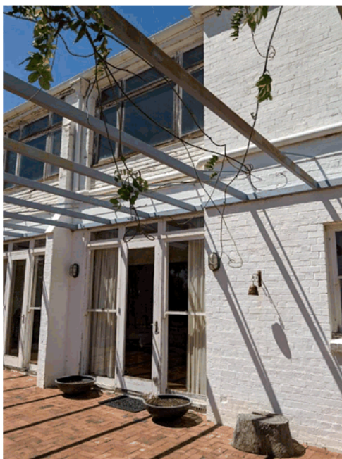
Figure 4 A close view of the outdoor terrace, dining room and the existing verandah above. Note the brick piers forming the verandah base, the weatherboard waist high first floor infills and the window panels: Two casement windows and a central fixed window with three matching fixed highlight windows above.
