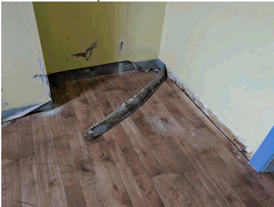
Image 24 Recommendations: Install damp course and desalination prior to new finishes
