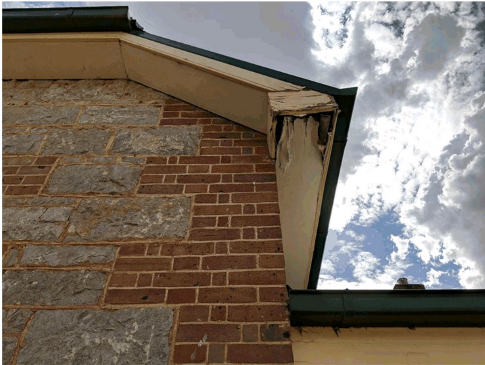
Image 2 Recommendation: Replace damaged eave with ventilated eave sheeting and finishing mould.
