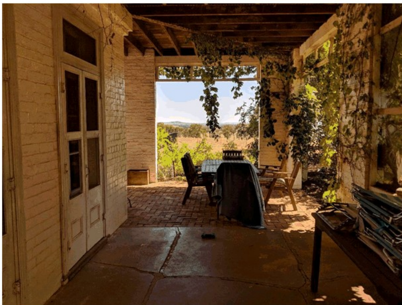
Figure 6 A general view of the front Eastern verandah, looking north, noting the external brick piers supporting the first floor verandah.
