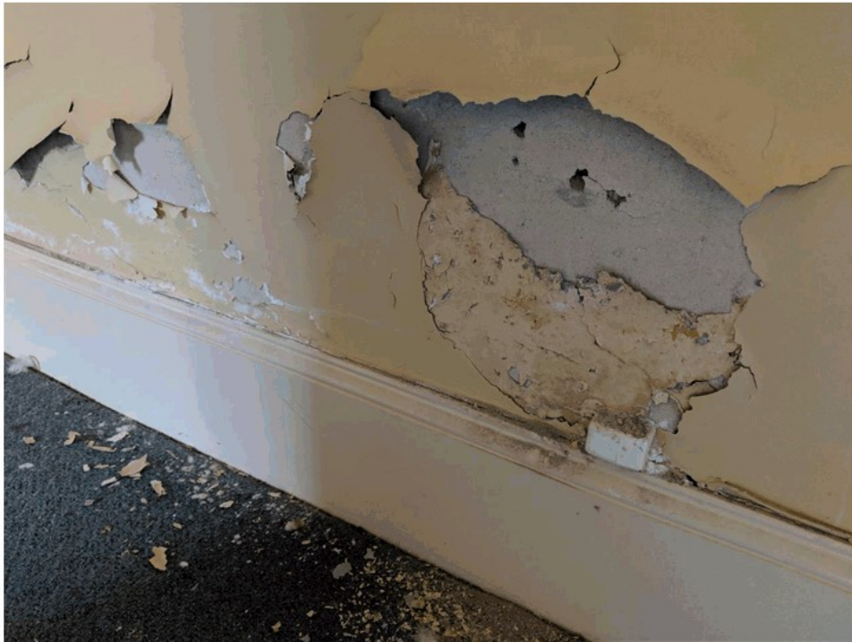
Image 28 Salt damp affected walls require new injection damp course and desalination to lower 900mm of wall render by Brad Asimus, Bathurst damp contractor 0263372624
