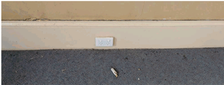
Image 30 Replace GPOs and switches with Tradco Heritage in antique copper Brown, toggle switches
