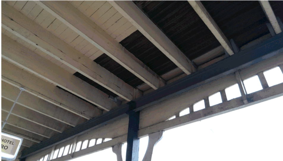
Figure 1 Note the perimeter bearer in a pfc section. This is a composite treatment where steel sections are applied like band-aids to an existing timber structure.
