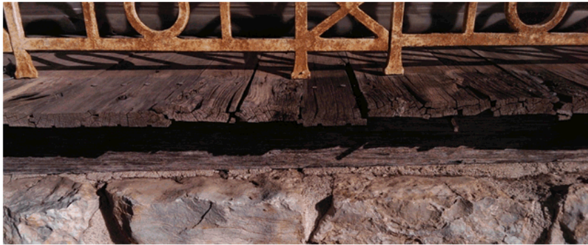
Photograph 6 Close view: The boards should have an external moulding to assist in supporting the outer edge fitted between the boards and bearer. As discussed two boards should be cut to align with the building and present an outer bull nose edge to increase the life of the timber.
