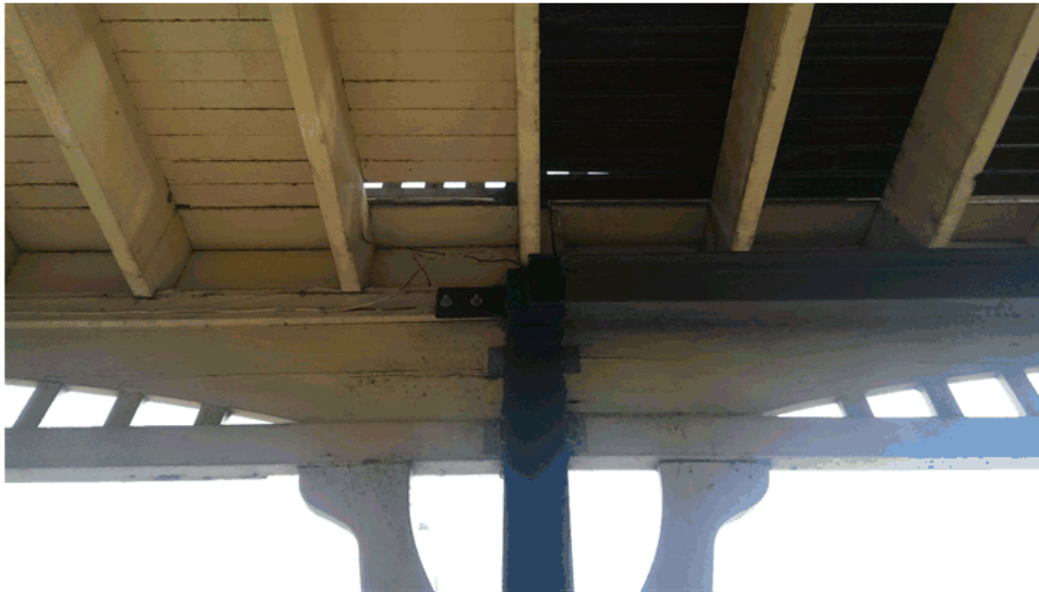
Figure 3 A detail view of the bottom section, the carved/shaped valence and the lower seating beam and upper bearer beam.
