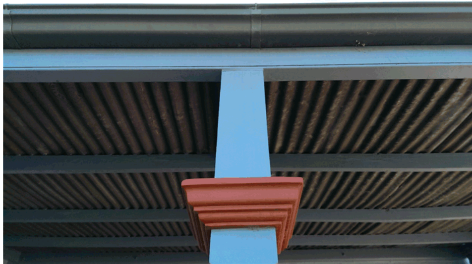
Figure 1 The fascia beam beneath the gutter would generally have been a different colour such as the Red to differentiate it from the posts and the gutter. This repeats the decorative elements seen on the post molds and the chamfers and generally gives the verandah additional vitality.
