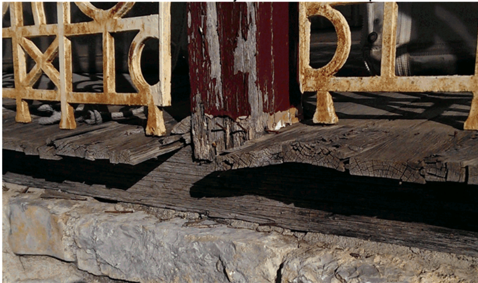
Photograph 5 Close view. The bearer should not be in contact with the mortar bed but have flashing or dpc to prevent moisture being drawn into it. As a rule, all the timber requires painting to preserve it. The cast iron elements will need to be removed, wire brushed, treated with Penetrol and painted.
