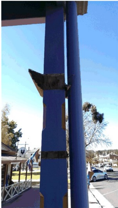
Figure 2 replacing the missing molds will complement the details. The reason it has failed is that the mold shape allows water to drain back against the post and rot the joints. The correct original mold profile would be formed to slope down from a high point where it fits against the post to the outer edge. This allows the water to run off and away from the joinery
