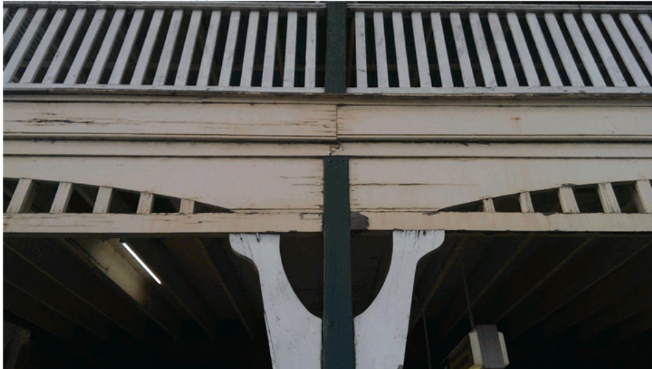
Figure 4 Detail view from the exterior looking at the members: The overall scope for a beam is a combination of the upper larger fascia section plus the smaller lower section which currently provides the seat for the joists.
