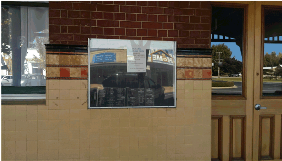
Photograph 36 The tiles were cut out for the sign. The sign could be re-fabricated to include a plaque on the bottom portion. This avoids affecting the original materials.
