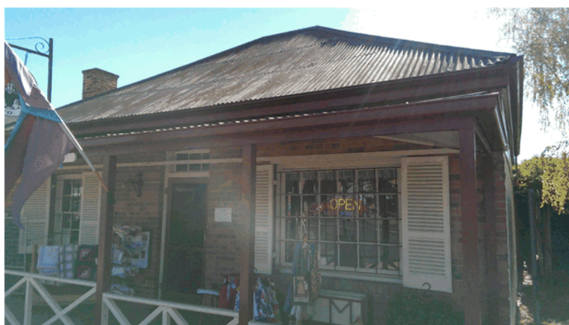
Figure 9 To seal the roof without losing the patina: A thorough pressure wash after a wire brush and then:
