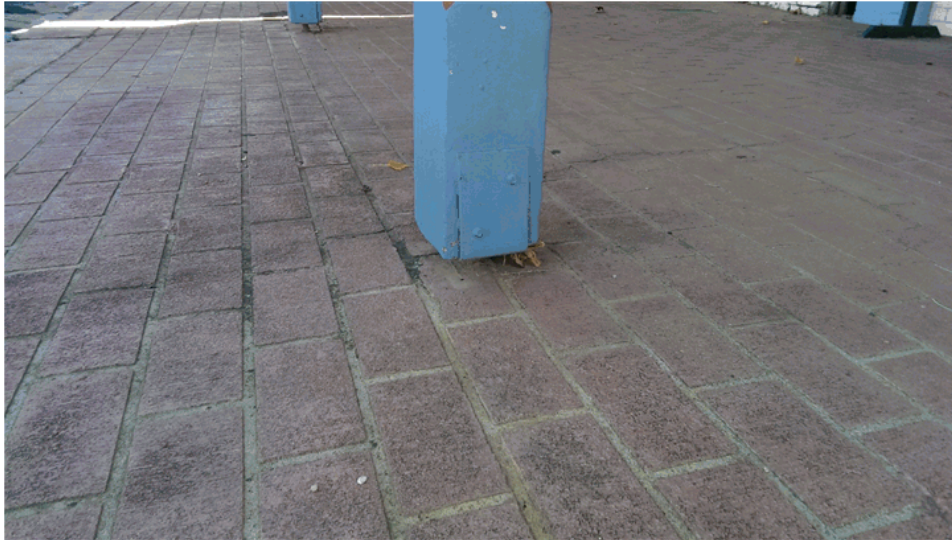
Figure 5 On a like for like basis it always looks best to place mitred skirting sections around the bases of the posts as this conceals the steel stirrups and bolts.
