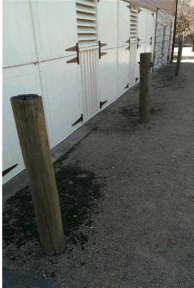
Figure 10 Hardware/ironmongery is always gloss Black with the correct fixings for timber. An alternate Cream would be fine on all the timber. Try cutting back to investigate the earlier colours as a Guide and speak with Catherine McKenzie at the Molong Museum to see what early photos she has as a guide.
