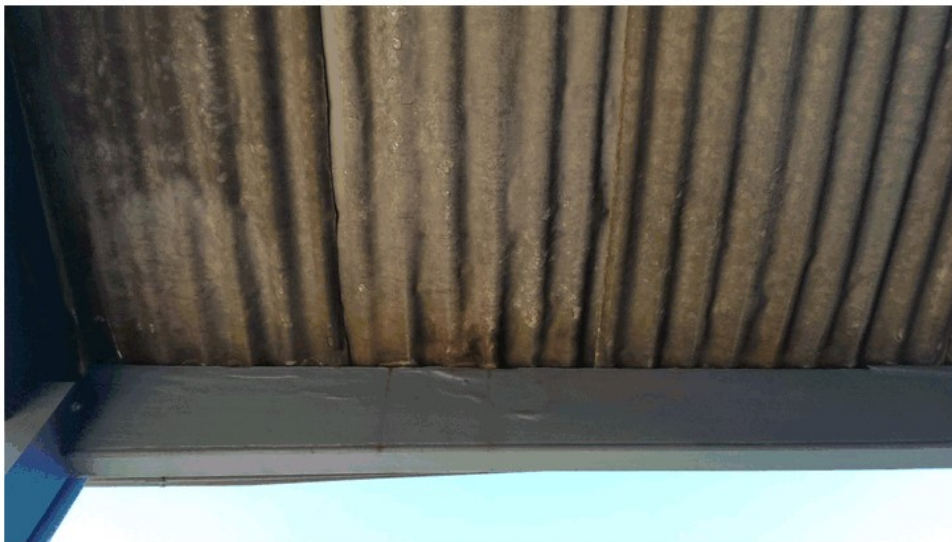
Figure 2 replacing the missing molds will complement the details. The reason it has failed is that the mold shape allows water to drain back against the post and rot the joints. The correct original mold profile would be formed to slope down from a high point where it fits against the post to the outer edge. This allows the water to run off and away from the joinery
