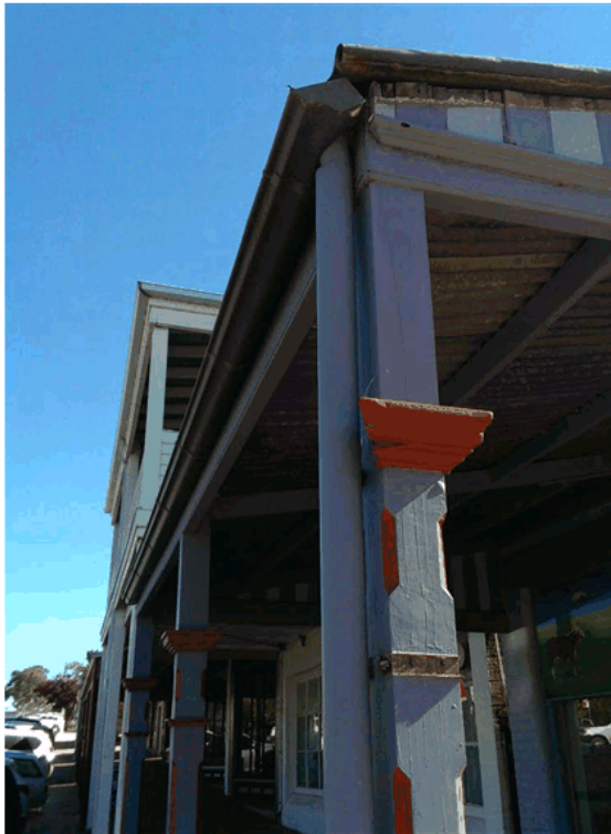
Figure 6 Missing molds as noted and end of the barge roll which requires a spear pint to make the water drip off the flashing.
