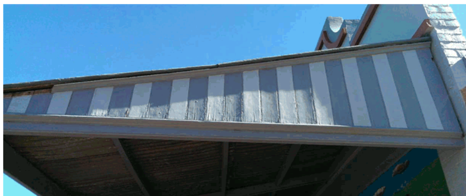
Figure 8 Replacing the boarding to match the existing including the under mold to the barge roll and lower mold to finish the boards would be fine – No need to match the other buildings. In colour terms the red would come back around the side on the fascia beam and complete the picture.
