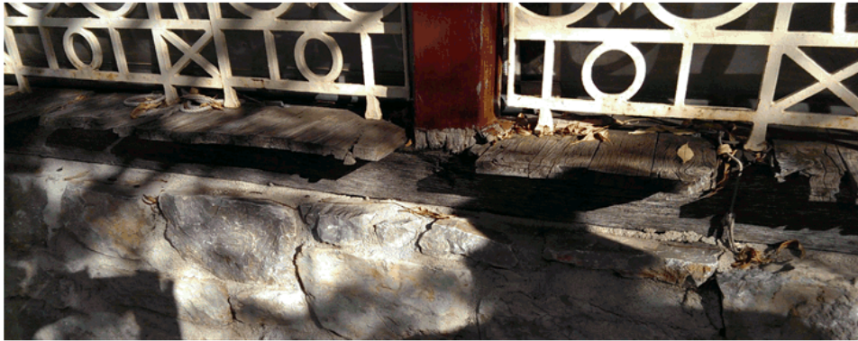
Photograph 4 Post damage requiring new bases to be spliced on to the existing where they are sound. The wall may require an additional capping course if the replacement bearer is relocated inwards. This is all subject to advice from an experienced builder.
