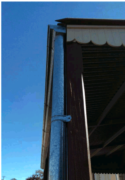
Figure 6 Missing molds as noted and end of the barge roll which requires a spear pint to make the water drip off the flashing.
