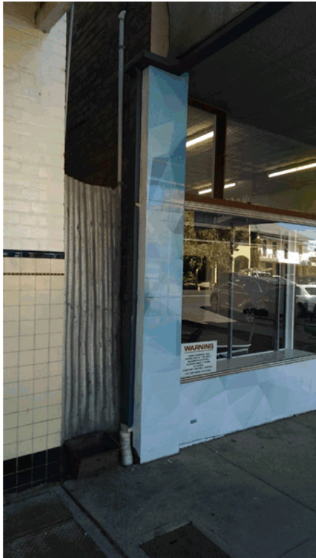
Photograph 28 The tiles are not original or significant. The colour scheme is vinyl overlay. This pier is not visually obstructive or replacing corporate images/signs.
