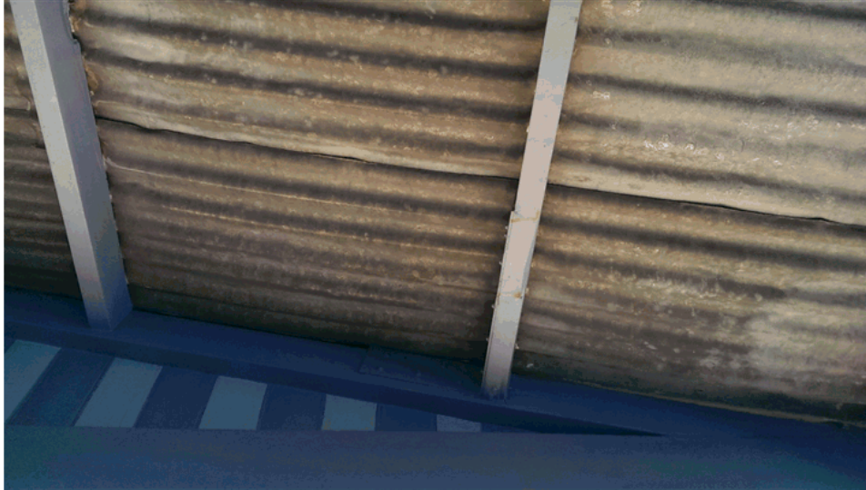
Figure 4 Note the damaged ends of the purlins and the possible rot from the ends of these purlins. Check the Framing code to ensure that the beam size and spacing meets the requirements. Note that the traditional colour for verandah soffit timber was Sage Green or similar. This could solve the problem of NOT having t match the blue colour.
