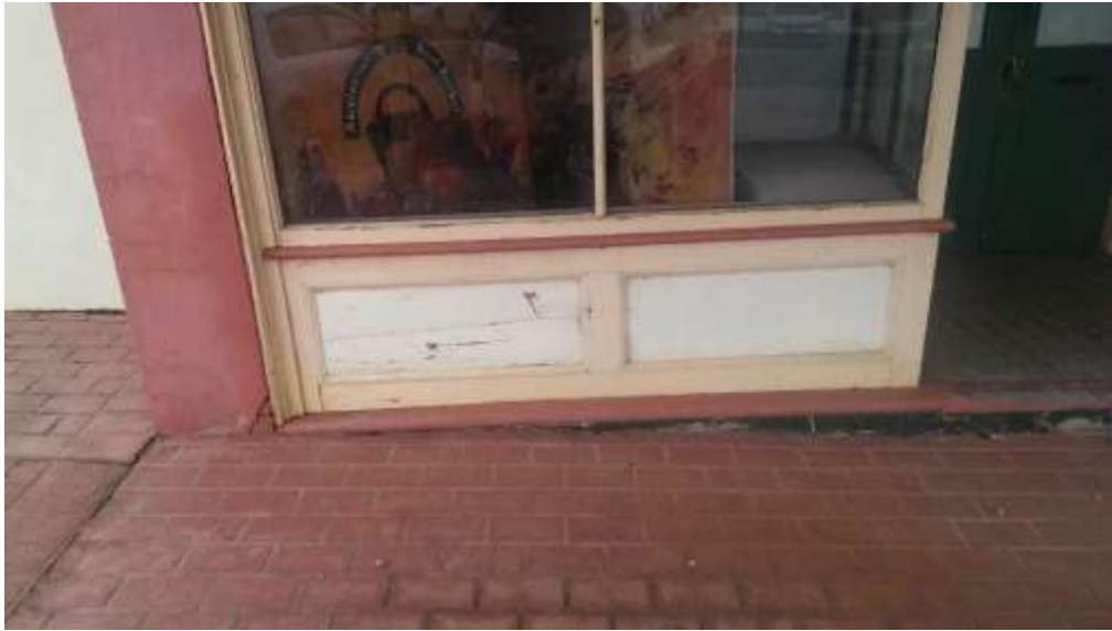
The base of the shopfront and rendered side pier
