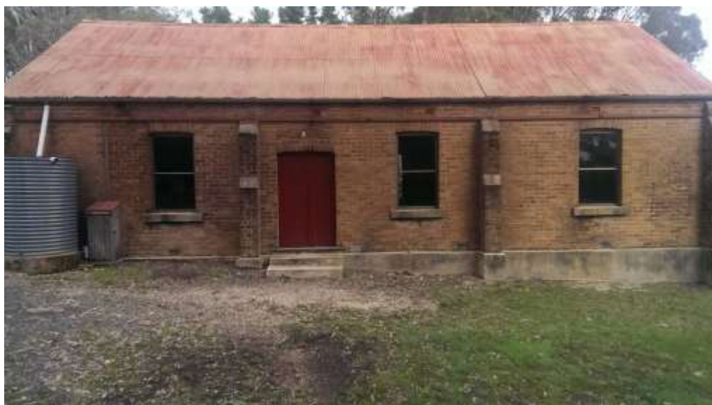
Similar situation along the north elevation. Note ground erosion and roof condition.
