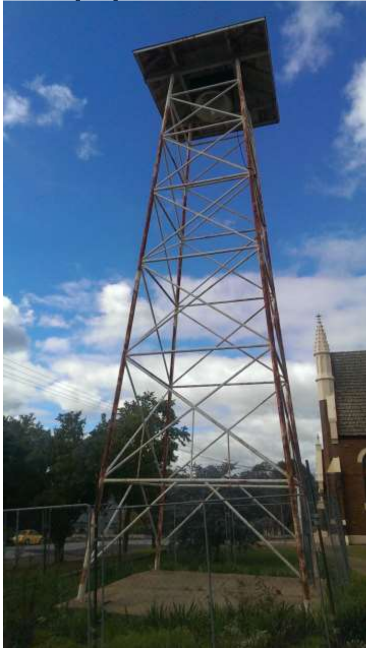
View of the tower. Notes the six frames and the tapering profile, the timber support frame, and the tin roof
