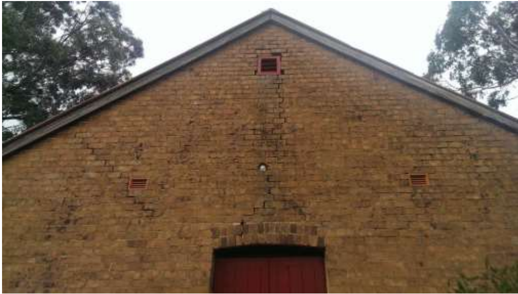
Movement causes cracking at the weak point in the west elevation
