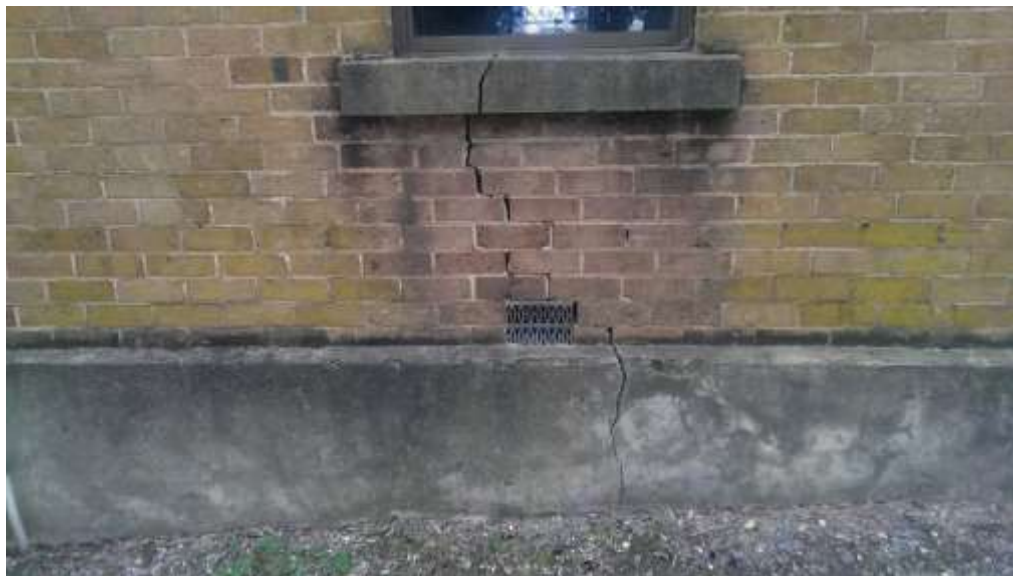
Typical crack caused by the ground shrinking at the south west corner
