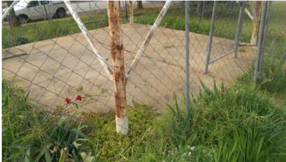
View of concrete base surrounding the steel frame and the temporary protective fencing.
