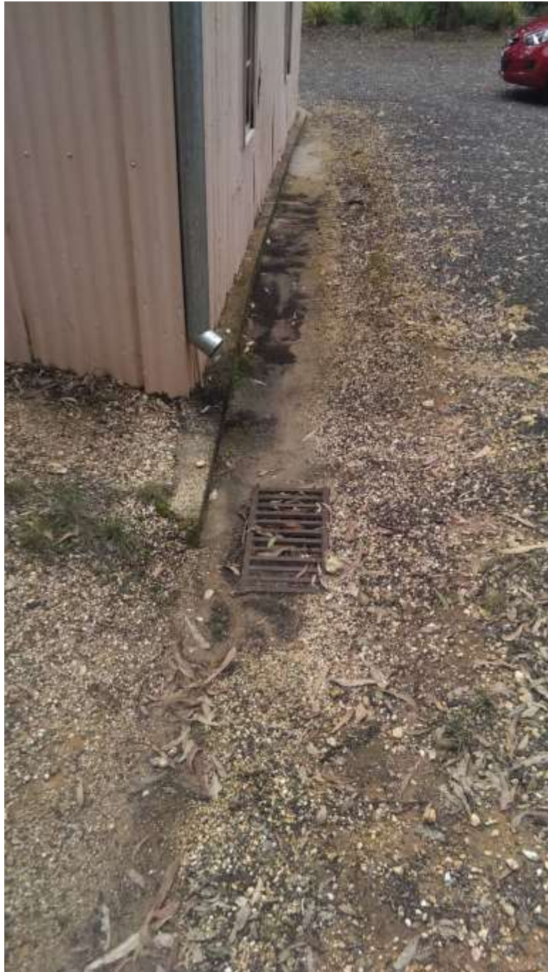
Note the damp ground due to poor water distribution along the rear of the hall
