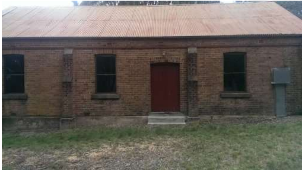
General North elevation: Brick piers and the steel section connecting the rods. The roof is in poor condition and replacement to be budgeted after inspection. Note surface erosion in the vicinity of the wall.
